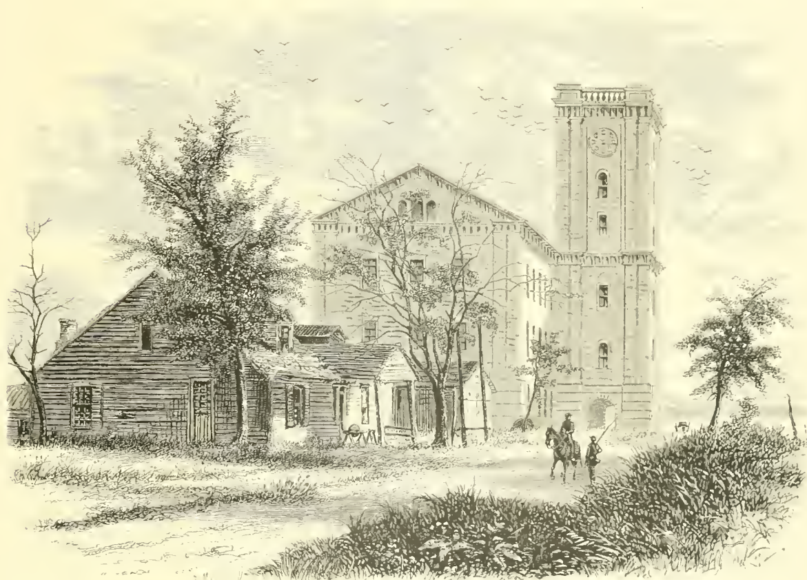
Old Arsenal, Rock Island.
